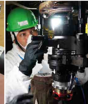
> On-site machining in a constricted environment subject to ionizing rays, achievable with a SERCO TU surfacing machine
