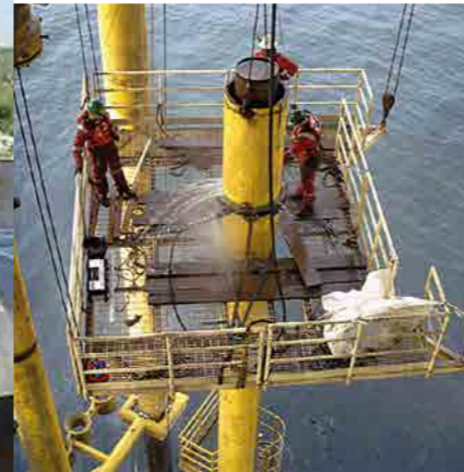
> Maintenance work on an oil platform using a PROTEM TT cutting machine
