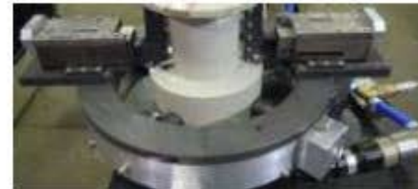
Coating removal with TTNG machine
